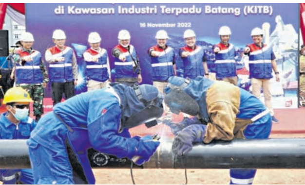
First welding infrastruktur distribusi gas bumi KITB.
